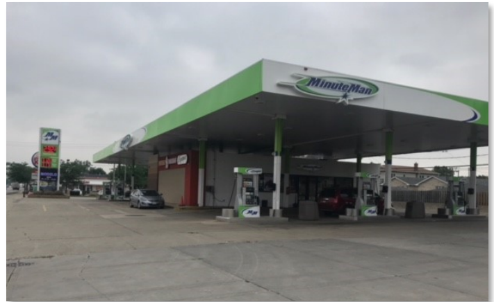
All three Chicagoland gas stations are now equipped with a fully integrated, innovative surveillance system
